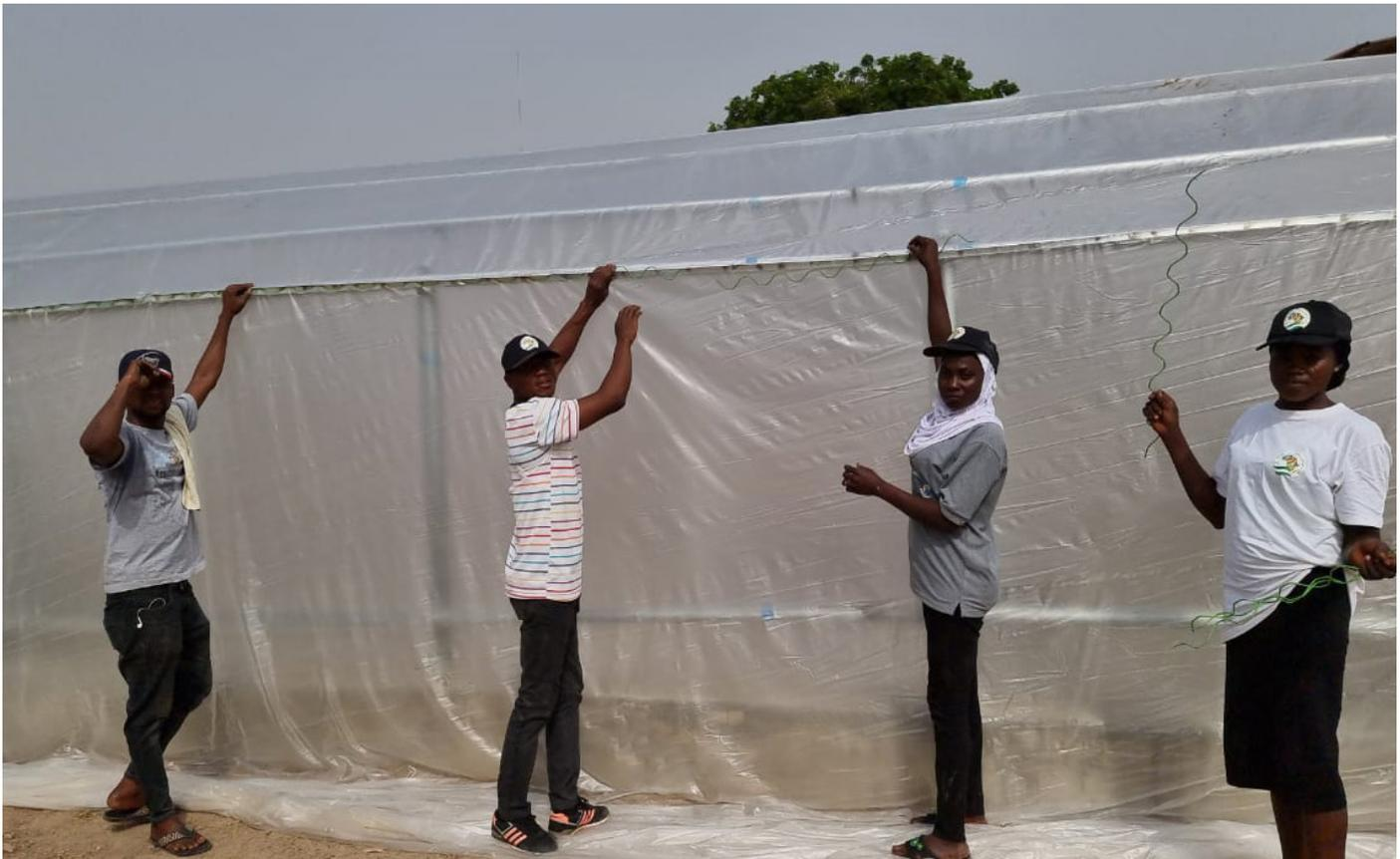
**EBAFOSA trained youth taking roles in building a solar dryer to help avert post harvest losses from the local community. The solar dryers are an inexpensive tools built to help drying of cereals and other leguminous produce. The drying allows the farmers to later add value to their produce and increase their shelf life.**
